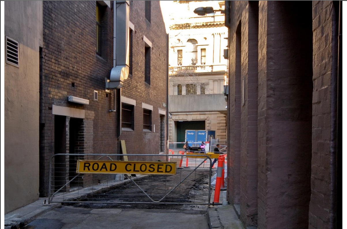
Market Row construction 2010
